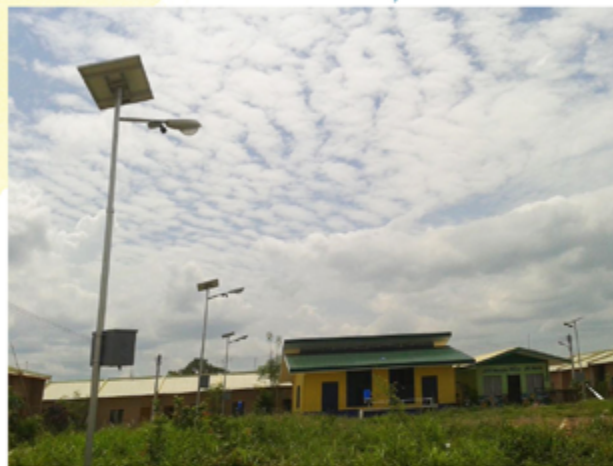
Solar-powered streetlights at Xavier Ecoville
